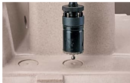
B - Place the drill aligned with the pre-punched hole
